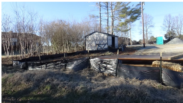
Expanded the Area with the Silt Fence February 25, 2025
