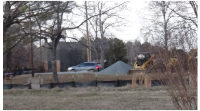
Adding Silt Fence and Gravel Base February 4, 2025
